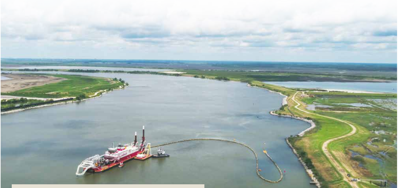
Deepening the inner harbor of the Savannah River. (Photo courtesy of Georgia Ports Authority)
